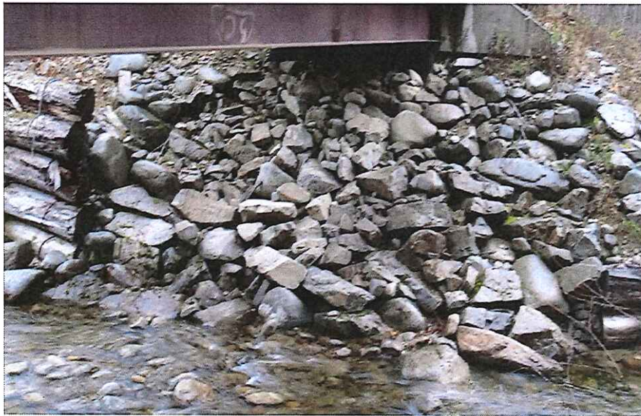
CK2296 Left Abutment
