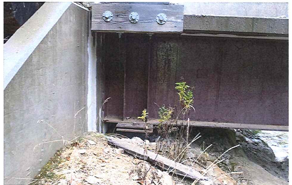
CK2296 Right Abutment bearing
